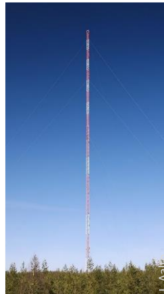
Instruments on mast (130m) and towers to measure at different heights
