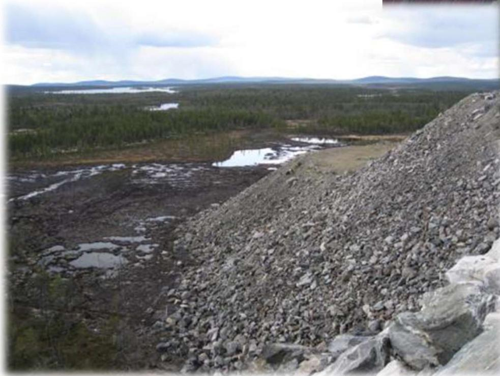
Total surface area of the waste dump is 33 ha, and the rock volume amounts to 6.7 million m<sup>3</sup>. The rocks of the dumping site represent overburden chiefly valueless gneisses, granite-gneisses, amphibolites and enclosing rocks mineralized to different extents: peridotites, olivinities, contact amphibolites, etc.
